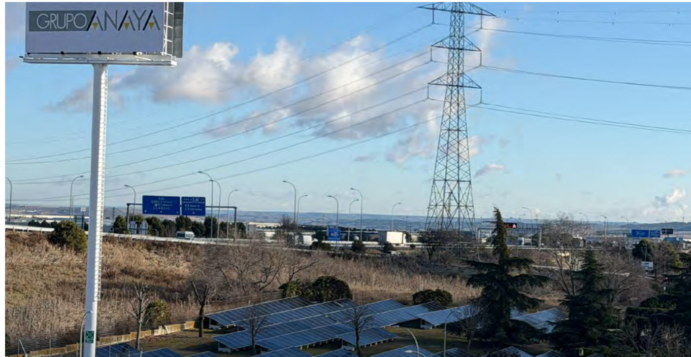
Installation of solar panels at the logistics site in Getafe, Spain (Grupo Anaya).
